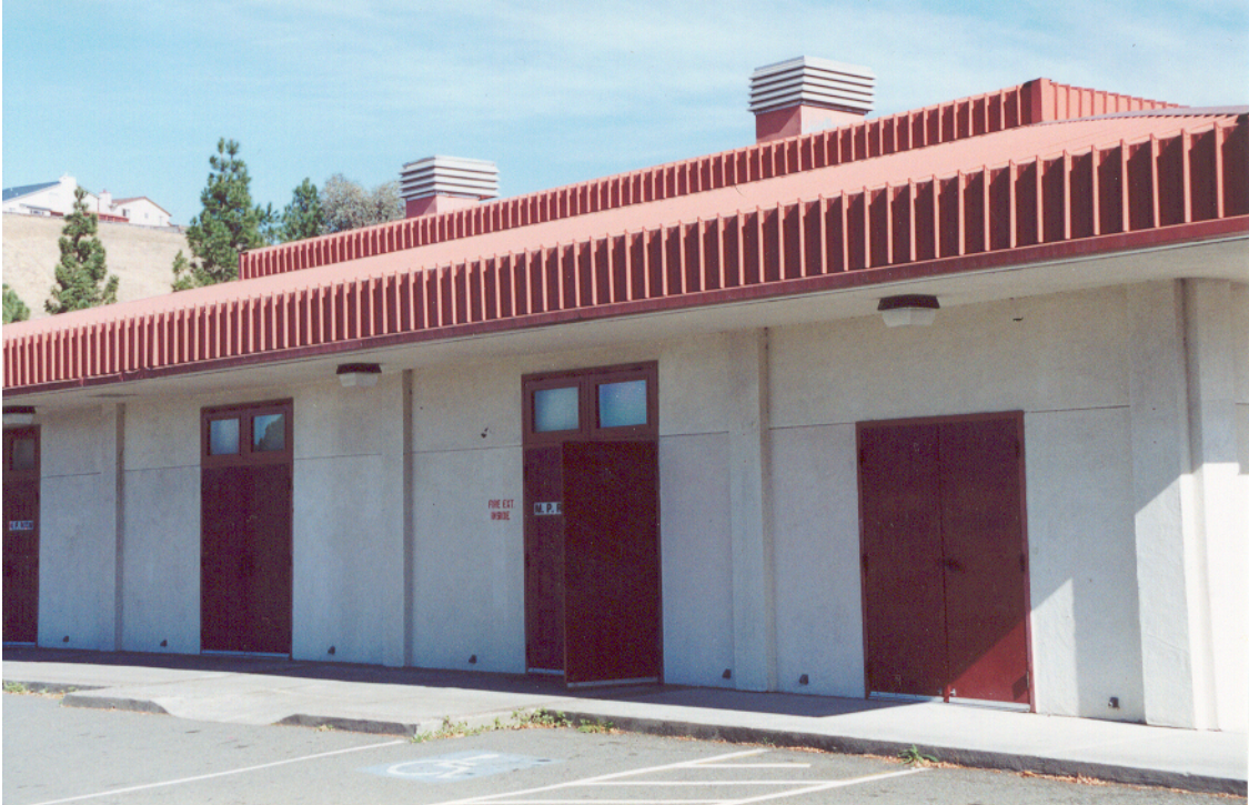
Figure 6: West Wall of Multi Purpose Building
