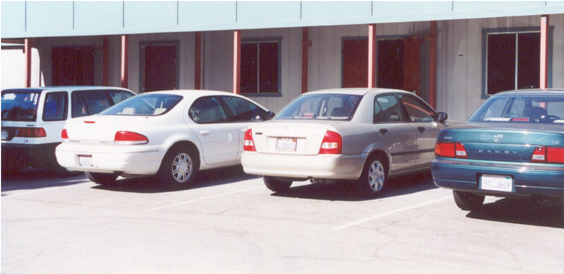
Figure 3: South wall of Administrative Building
