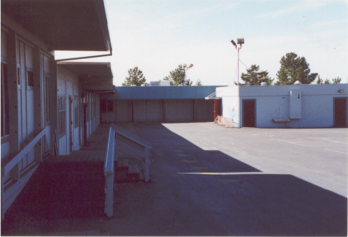
Figure 5: North Wall of Original Classroom building (Room numbers 1 through 4)
